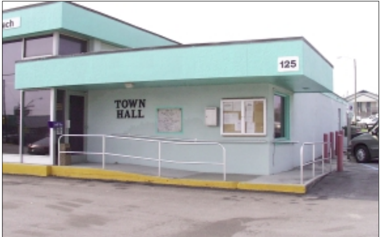
An accessible route connects accessible parking (right) with the accessible entrance.
