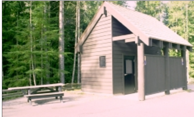
Public toilets at a park were built to comply with the new construction requirements of the ADA Standards.
