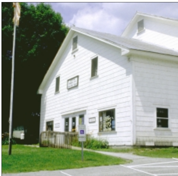
Alterations to existing town buildings follow the alteration requirements of the ADA Standards.
