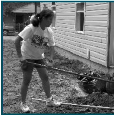
HN Marilyn Ongoco levels the yard at the yard at Habijax.
