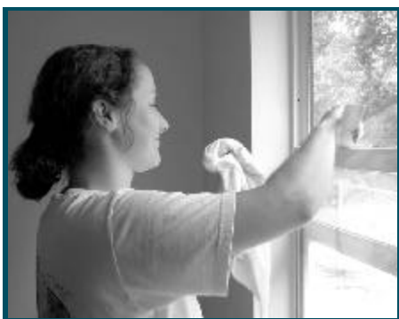
HM3 April Halberg prepares a window surface before painting.
