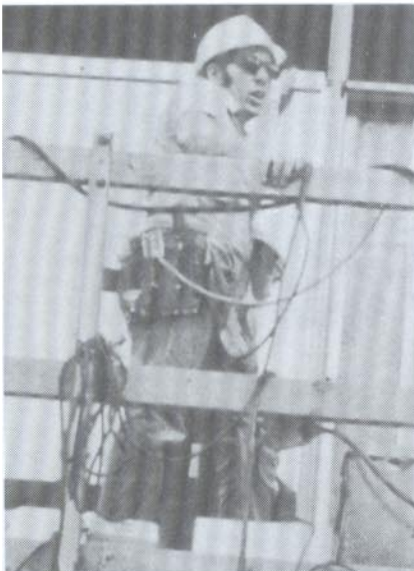
Worker with fall protection systems in place.
