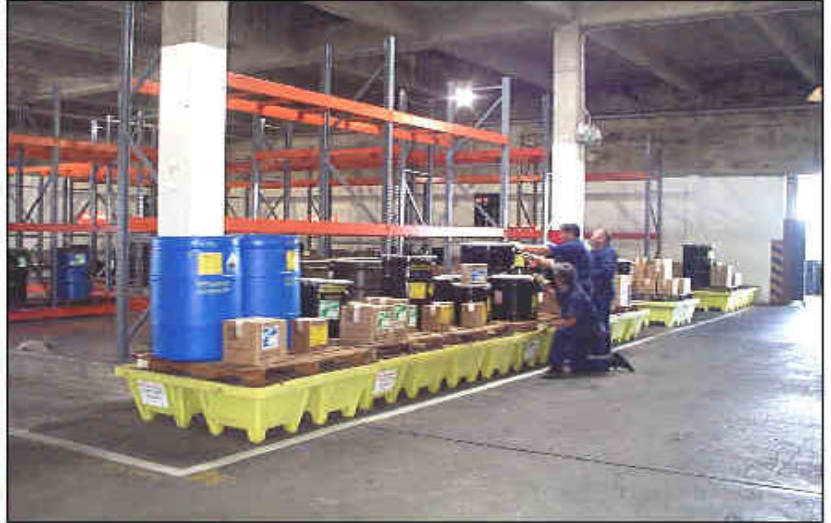
Building 229, HAZMIN Center
