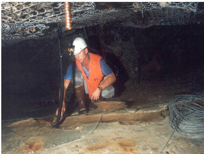
Figure 9.—Thrust-fault-type failure, November 4, 1997.
