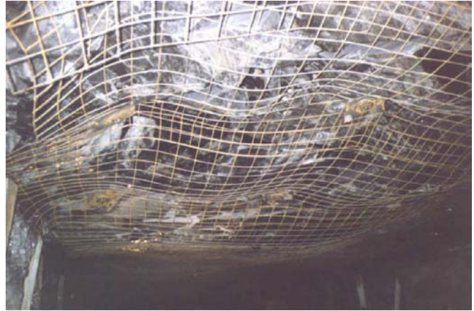
Figure 29.—Metal screen supporting roof scale formed in highly slickensided shale.
