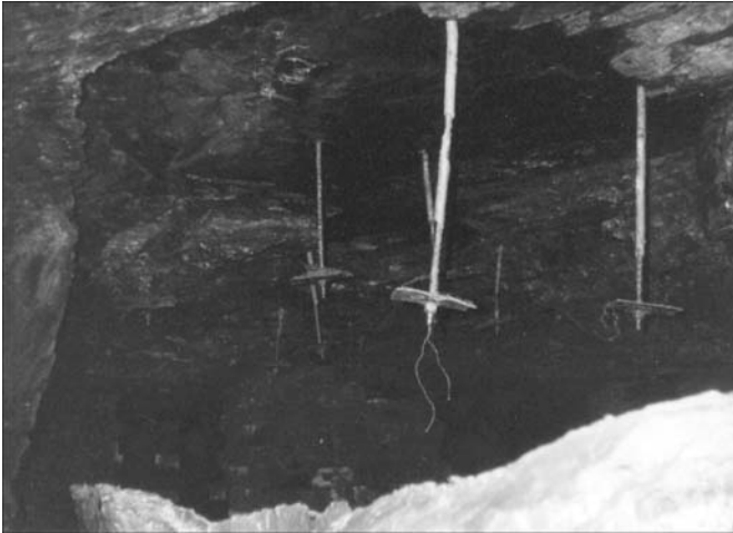
Figure 45.—Roof fall caused by broken rock falling between bolts.
