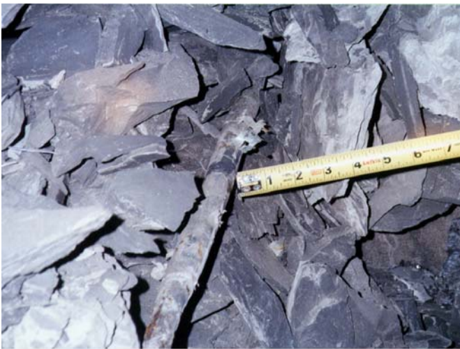
Figure 45.—Roof fall caused by broken rock falling between bolts.
