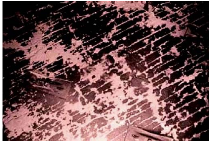
Figure 35.—Systematic jointing in the shale roof of a southwestern Pennsylvania mine continued only about 6 in vertically and terminated against a siltstone.
