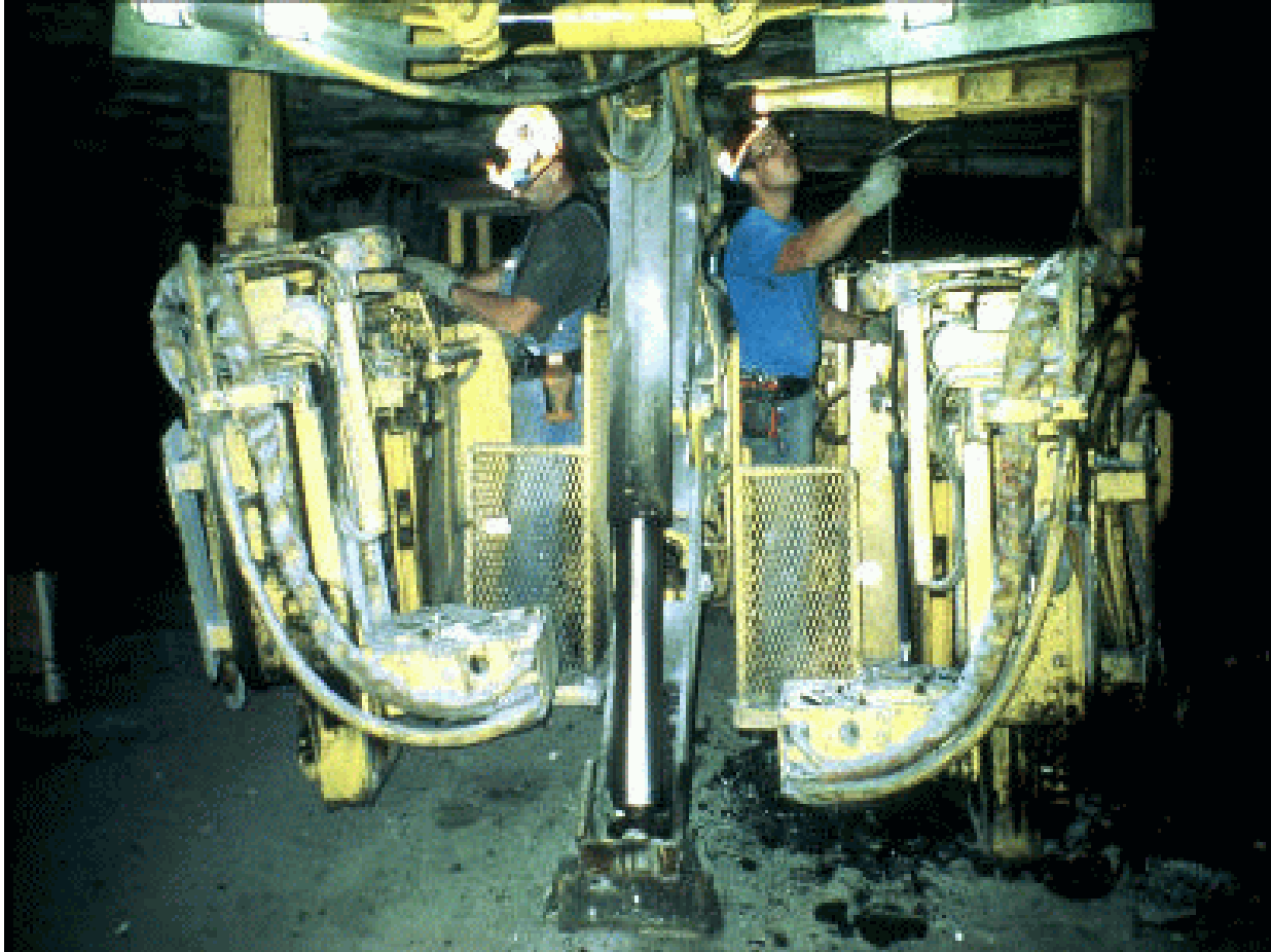
Figure 2. Workers roof bolting in a high seam mine.
