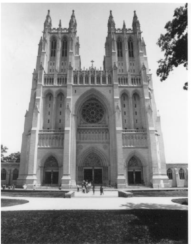
Figure 2. View of the west front and west wings of Washington National Cathedral.
