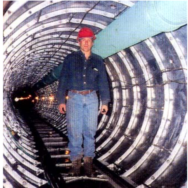
Figure 1. Steel liner plate commonly used to provide temporary lining of tunnels.
