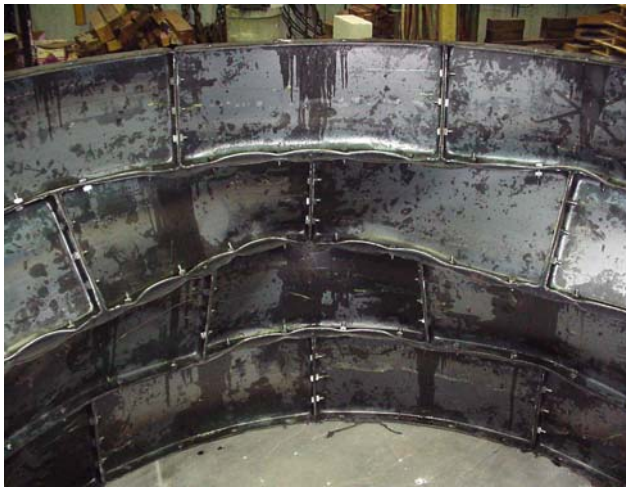
Figure 11. Middle two rings controlled the failure of the four-layer configuration.
