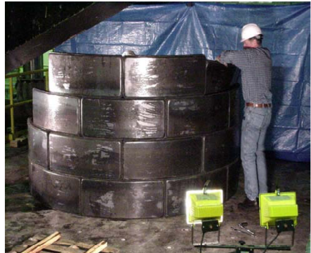
Figure 3. Four layer section of liner plate being constructed in the Mine Roof Simulator for full-scale testing.
