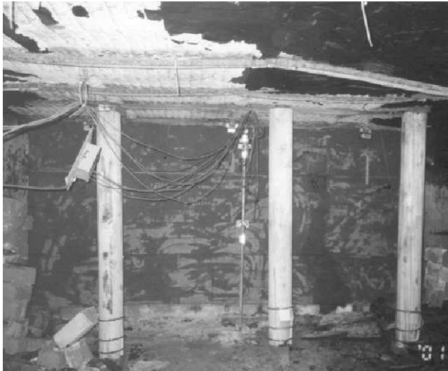
Figure 3. Photo of the replacement stopping at 33 crosscut
