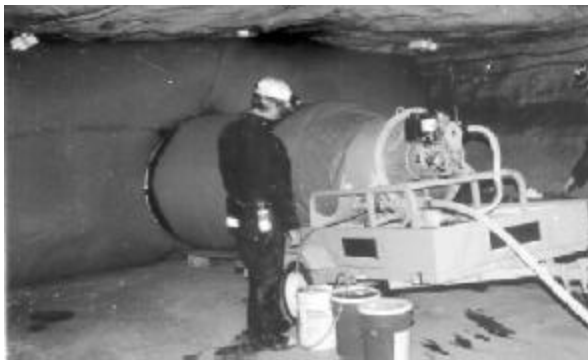
Figure 8 - Photo of inflatable feed-tube partition in the Lake Lynn Experimental Mine.
