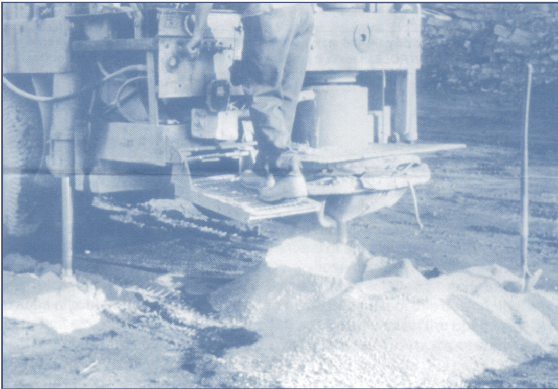
Figure 2. Drill operator at the control panel.
