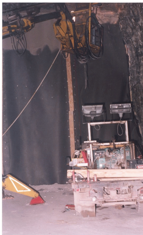
Figure 8. Fabric-grid material sprayed with cementitious material.
