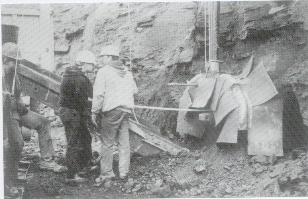
Figure 1.—Inert gas shroud enclosure of auger hole collar. Note small-diameter pipe used for collar measurements.
