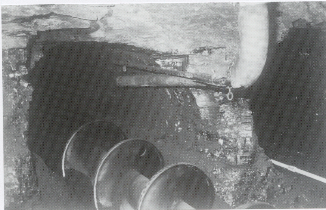
Figure 2.—Inert gas stub pipe used to direct inert exhaust into the hole. Note small-diameter pipe used for collar measurements.
