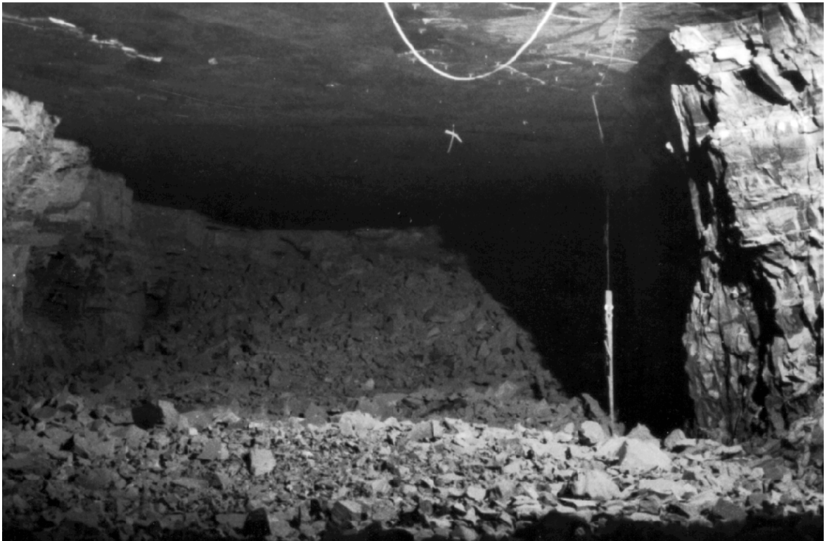
Figure 16.—Mine face after blast 6, showing rubblization. (Photo by Kenneth L. Cashdollar, Pittsburgh Research Center.)
