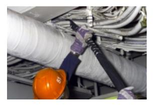
The rope is attached to the cable with a wire mesh-pulling grip and is threaded
