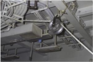
The NNSY study team engineered a mechanically assisted cable pulling process that reduces the potential for injury to personnel and requires less time and effort. It uses a cable-pulling winch (capstan), double braided low stretch rope, pulleys, and Teflon sheets to reduce cable friction.
