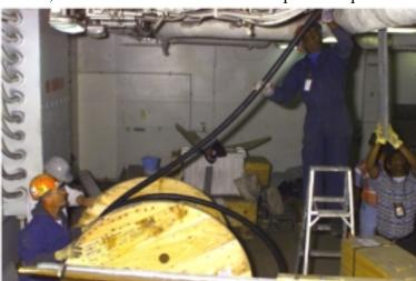
days. Initial tests aboard USS SAIPAN and USS NASSAU indicate a potential for reducing cable pulling time and costs by as much as 50% with no personnel injuries. The initial test runs resulted in a combined savings to the Navy of over \$118,000. Projected future savings will vary from ship to ship depending on the length of the cable run.
