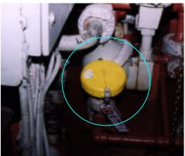
power source, providing a positive barrier between the power source and the person working on it. The only individual authorized to remove a lock or tag, is the person who installed it. In an emergency, the ship's Master or Chief Engineer may remove a tag or lock, <u>only</u> after verifying to ensure that no one would be adversely affected by reenergizing the system.
