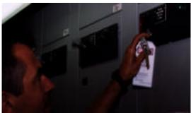
Lockout/Tagout Program reduces that risk of personal injury and property damage. Since equipment and machinery power sources come in many forms, there are situations when it isn't feasible to attach a lockout device and lock. In those cases, a tagout system alone must be used.
