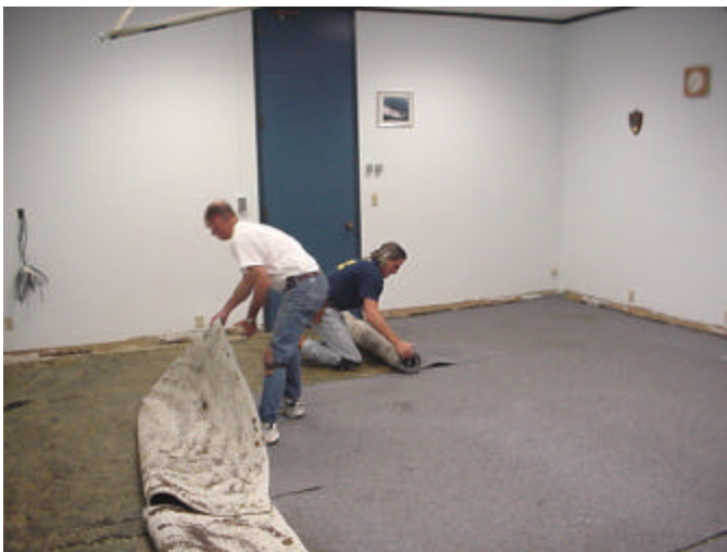
Workers had to kneel, squat, and stretch over long periods, which added to strain on their backs and knees during carpet removal
