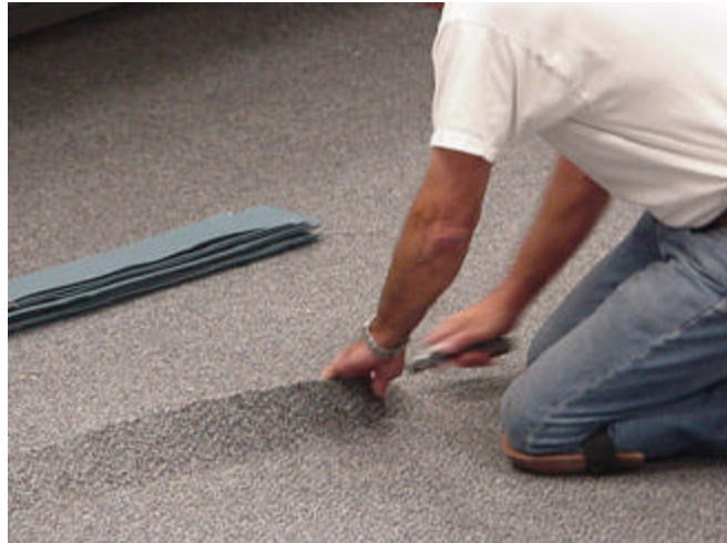
Maintenance workers used to kneel while removing carpet with a pinch-type gripping tool
