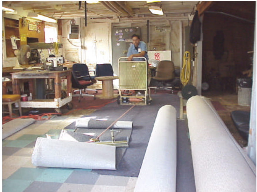
One worker, standing upright, removes a carpet, using a mechanical carpet puller
