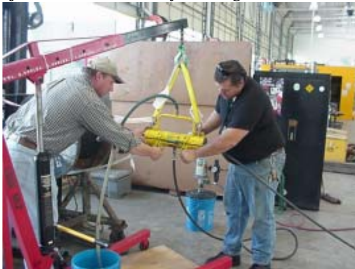
Crane riggers place the end of a wire rope into the automatic cleaning and lubrication system
