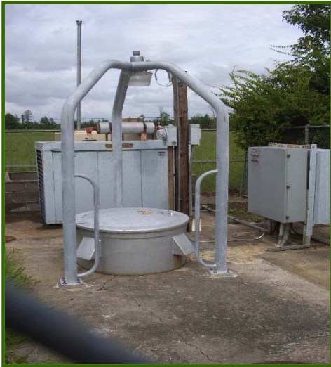
After: Stable rescue system anchorage.
