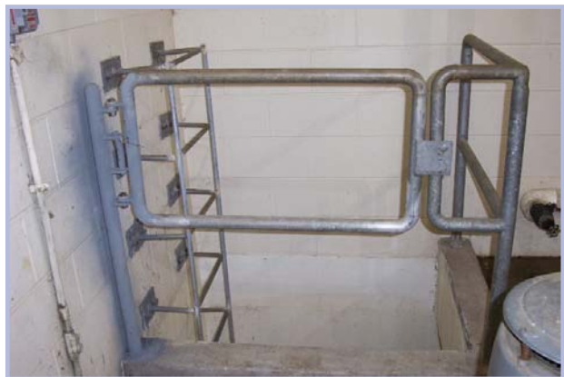
After: Self-closing swing gate on platform and vertical handrails on ladder.
