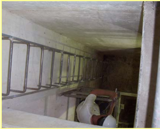
Installation of self-closing swing gate.
