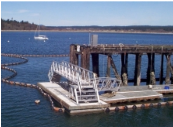
Floating dock with hydraulic winch
