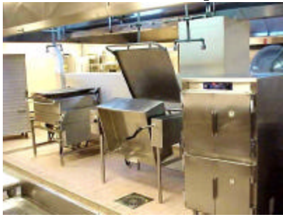
Bermed deep fryer area controls leaks and spills
