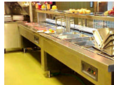
Self-actuating cart at left. Serving countertop at ergonomically correct height of 36 inches
