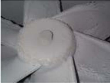
**Over 25 pounds of paint residue were removed from fan blades and ductwork**
