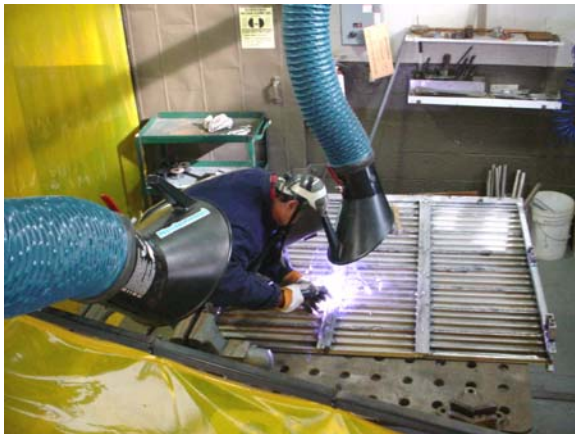
One of two flexible arms on air extraction unit is placed directly over welding area. Second arm (foreground) is available for use by another welder.
