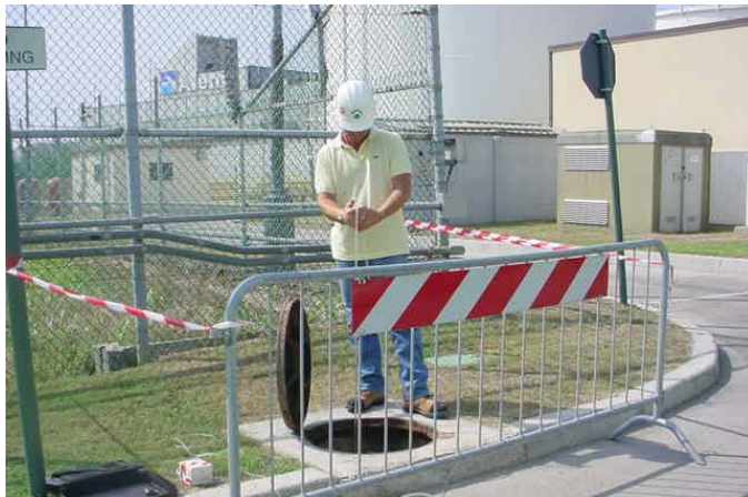
At NSA Naples, confined spaces are certified free of harmful gases before entry.
