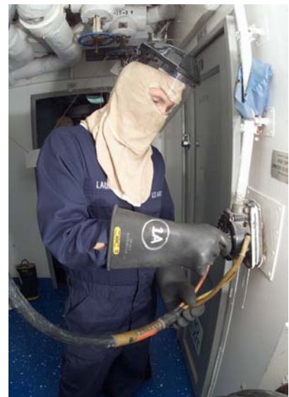
Interior Communications Electrician Fireman rigs a casualty power cable during a General Quarters Battle Drill scenario.
