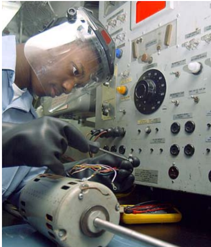
Electrician's Mate measures the resistance of a fan coil unit motor.
