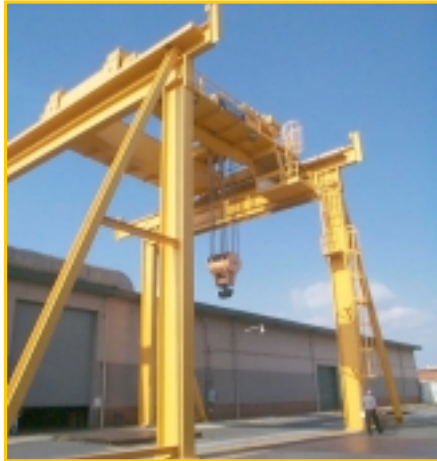
NAVICP's 60-foot high 400-ton bridge crane
