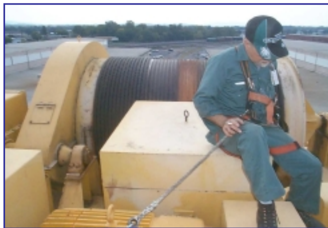
One anchor point for fall arrest gear resulted in very limited working area
