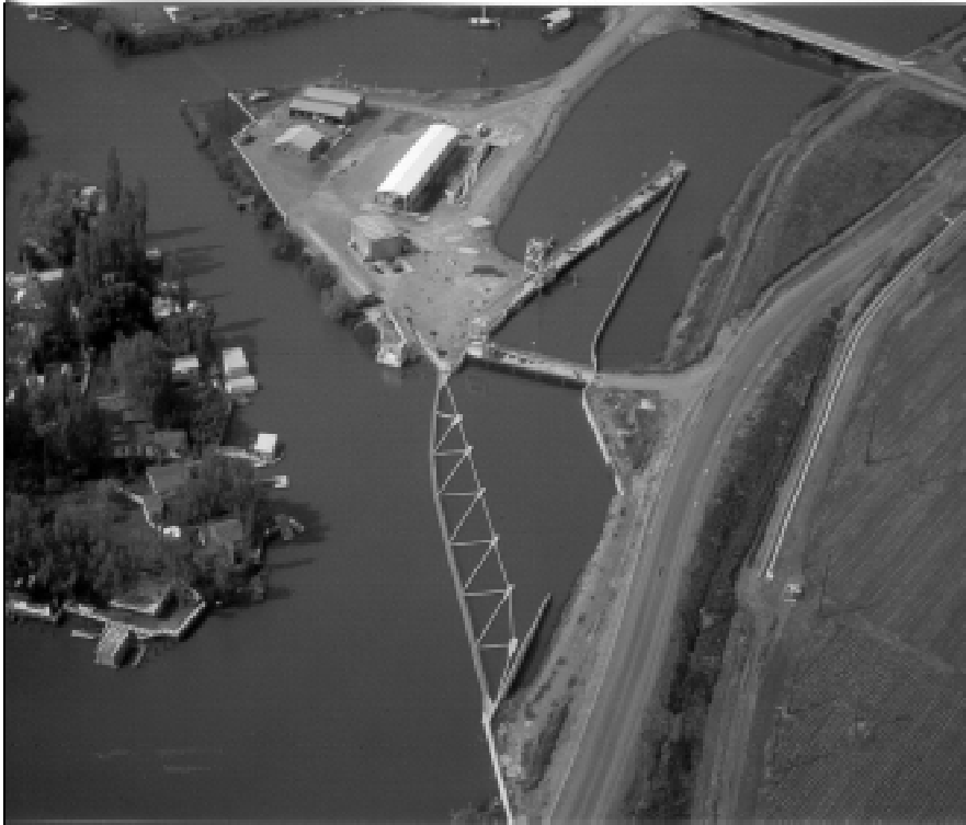
Tracy Pumping Plant and Fish Facility.
