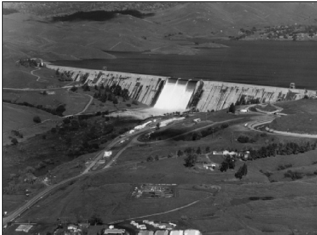
Friant Dam drum gates were replaced with crest gates in FY 1998.
