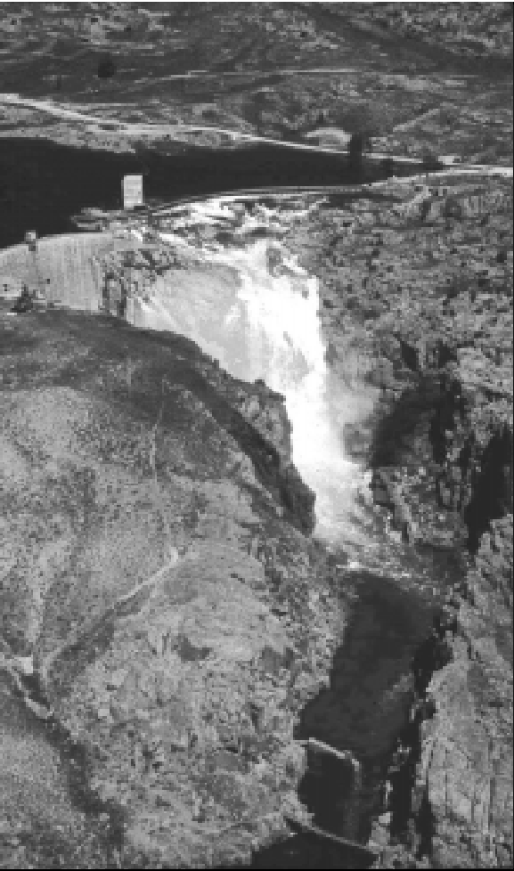
Pathfinder Reservoir on the North Platte River in Wyoming is a Reclamation facility that affects endangered species downstream in Nebraska.
