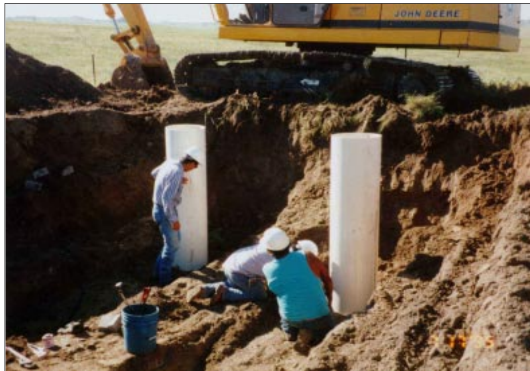
Construction of Mni Wiconi rural water project in South Dakota.
