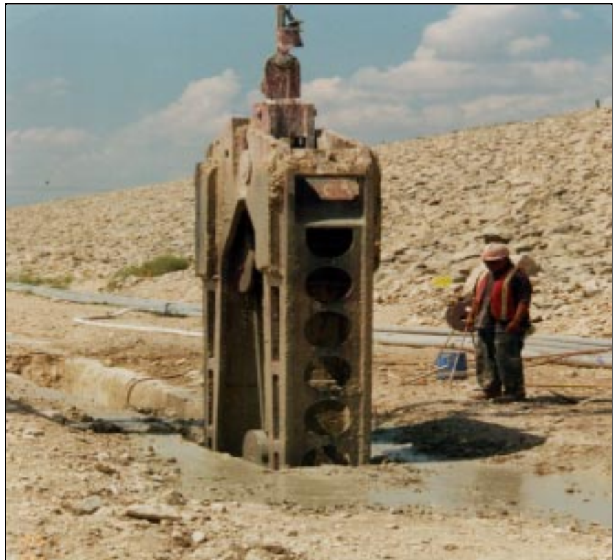
Safety of dams modifications underway at Twin Buttes Dam, Texas.
