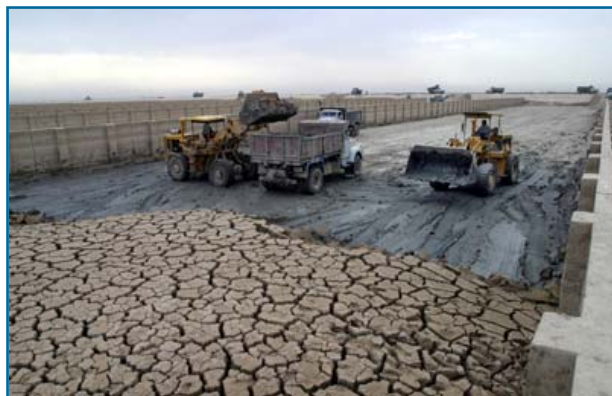
Above: Loaders remove accumulated silt from a Sweet Water Canal storage reservoir.
