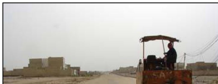
Street paving in a city in An Najaf Governorate
