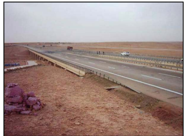
The newly rehabilitated Al Mat Bridge was reopened on March 3. Photo: USAID
