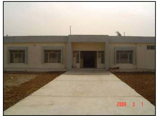
Newly renovated Basta Piazza Children's Center in Arbil. Photo: USAID
