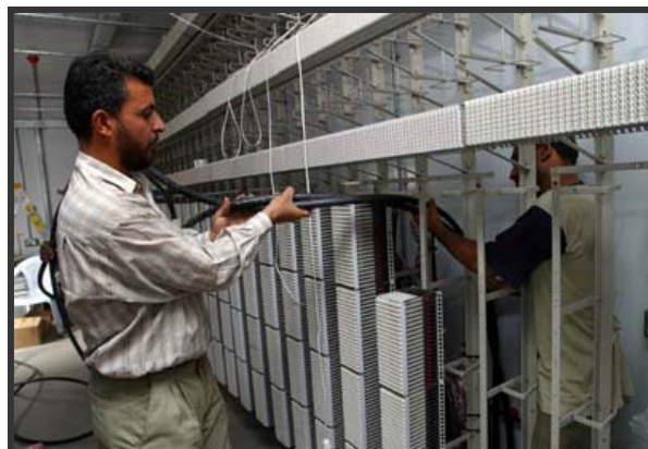
The Al-Mamoun Telephone Exchange where repair work will restore telephone services to approximately 30,000 subscribers. (Photo: Thomas Hartwell)
