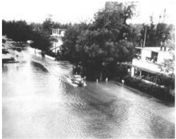
Flooding at Midway Island from the 1952 Tsunami (U.S. Navy Photograph)
