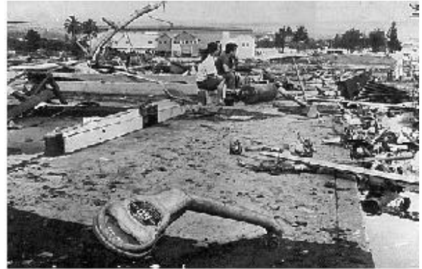
May 22, 1960. Tremendous force of tsunami waves and debris bent parking meters and snapped utility poles at Hilo, Hawaii. (U.S. Navy)
