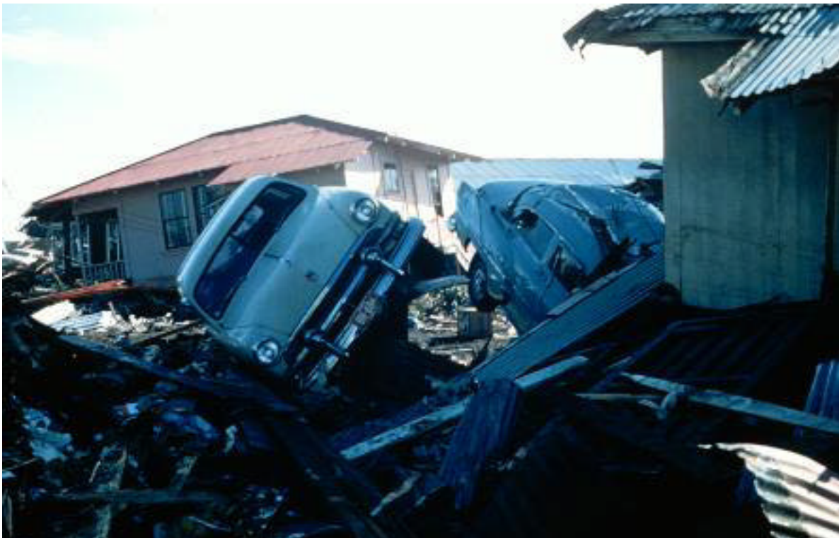
Photos of tsunami destruction of Hilo's waterfront
