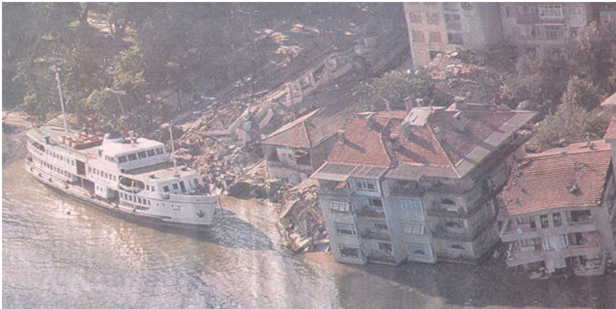
Subsidence and permanent flooding at Degirmendere, Turkey.
