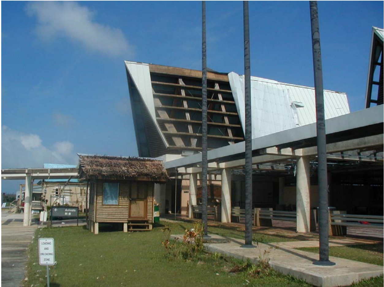
Figure 10. Yap Airport four days and much cleanup after Typhoon Sudal.
