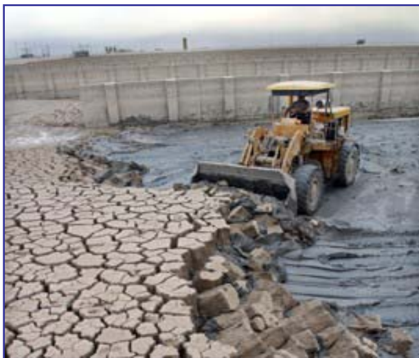
Above: Loaders remove accumulated silt from a section of 1 of 2 storage reservoirs in the Sweet Water Canal project that supplies all the fresh water to the city of Basrah and environs. When completed it will serve 1.75 million citizens of the Basrah region. (Thomas Hartwell)
