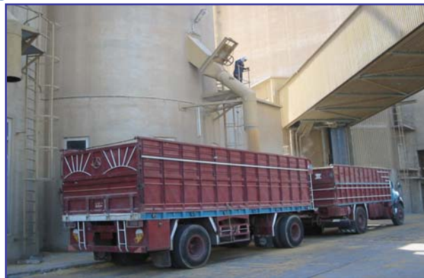
A recent shipment of grain to Umm Qasr port is being loaded onto trucks for delivery after being transferred into the newly restored grain silos. (Bechtel Photograph)
