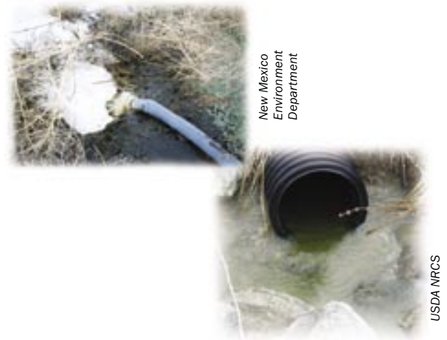
A pipe or ditch that carries wastewater to a stream is a discrete conveyance.
