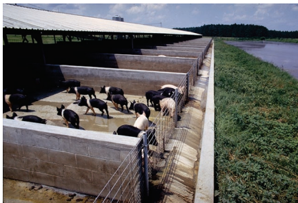
Hog parlor with a concrete floor and a conveyance that carries manure and wastewater to a lagoon.
