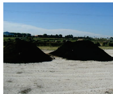
Runoff from unprotected stockpiles could pollute surface water.
