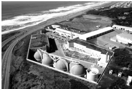
San Francisco's CSO Oceanside Water Pollution Control Plant treats an average of 17 million gallons per day (mgd) during dry weather and has 65 mgd of peak flow capacity.
