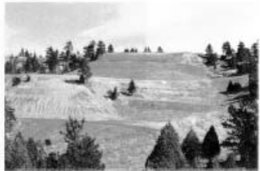
C. Slope reduction and installation of waterbreaks completed
