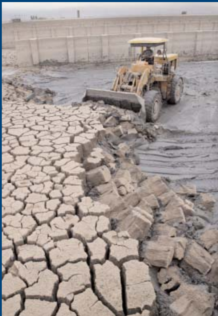
Removing caked silt from Sweet Water Canal reservoirs. The Canal system supplies water to 1.75 million people in Basrah governate.
