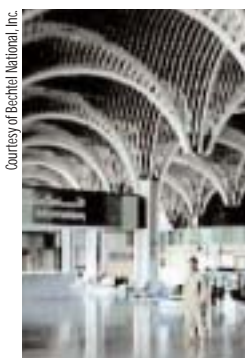
Reconstructed terminal at Baghdad International Airport
