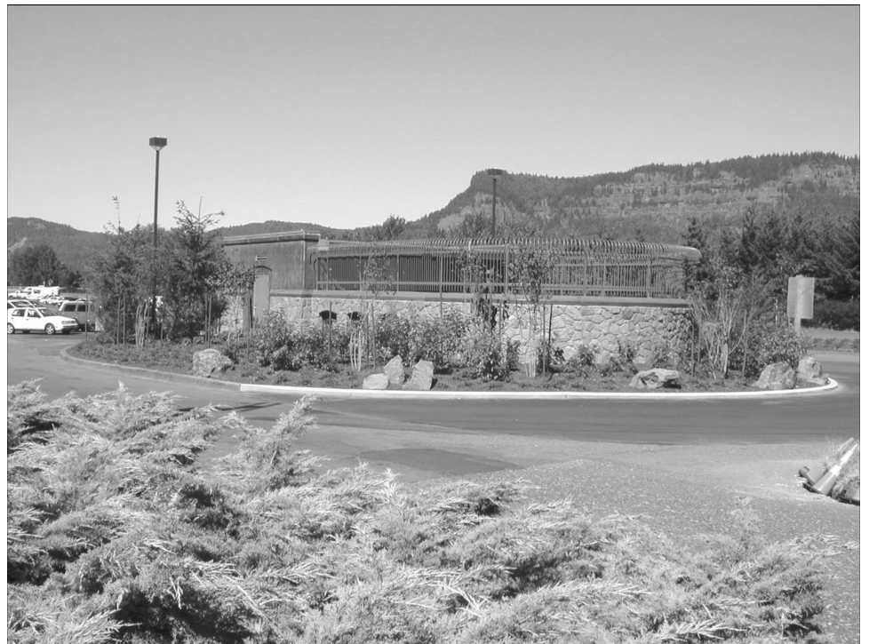
Figure 5: Wastewater Treatment Plant at Multnomah Falls
