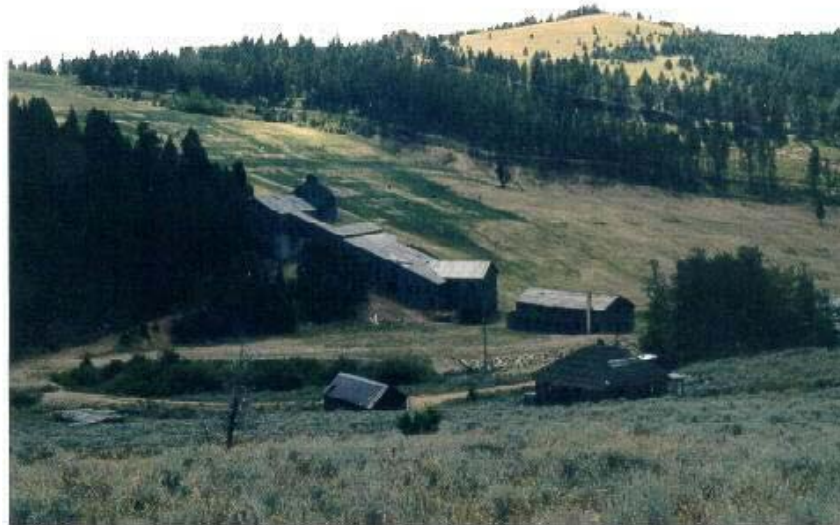
Comet Mine/Mill and part of the ghost town of Comet. Revegetated slope behind the old mill structure was once a huge open pit.
