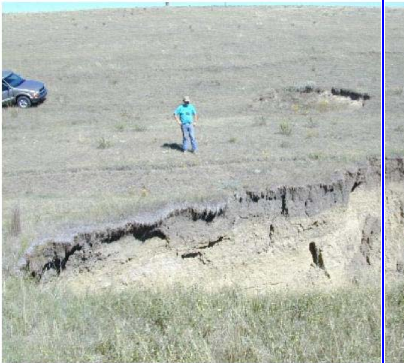
This sinkhole was located on pasture land owned by Mike Wolf near Dickinson. 65 cubic yards (equivalent to 65 truckloads) of dirt were needed to fill this hole.
