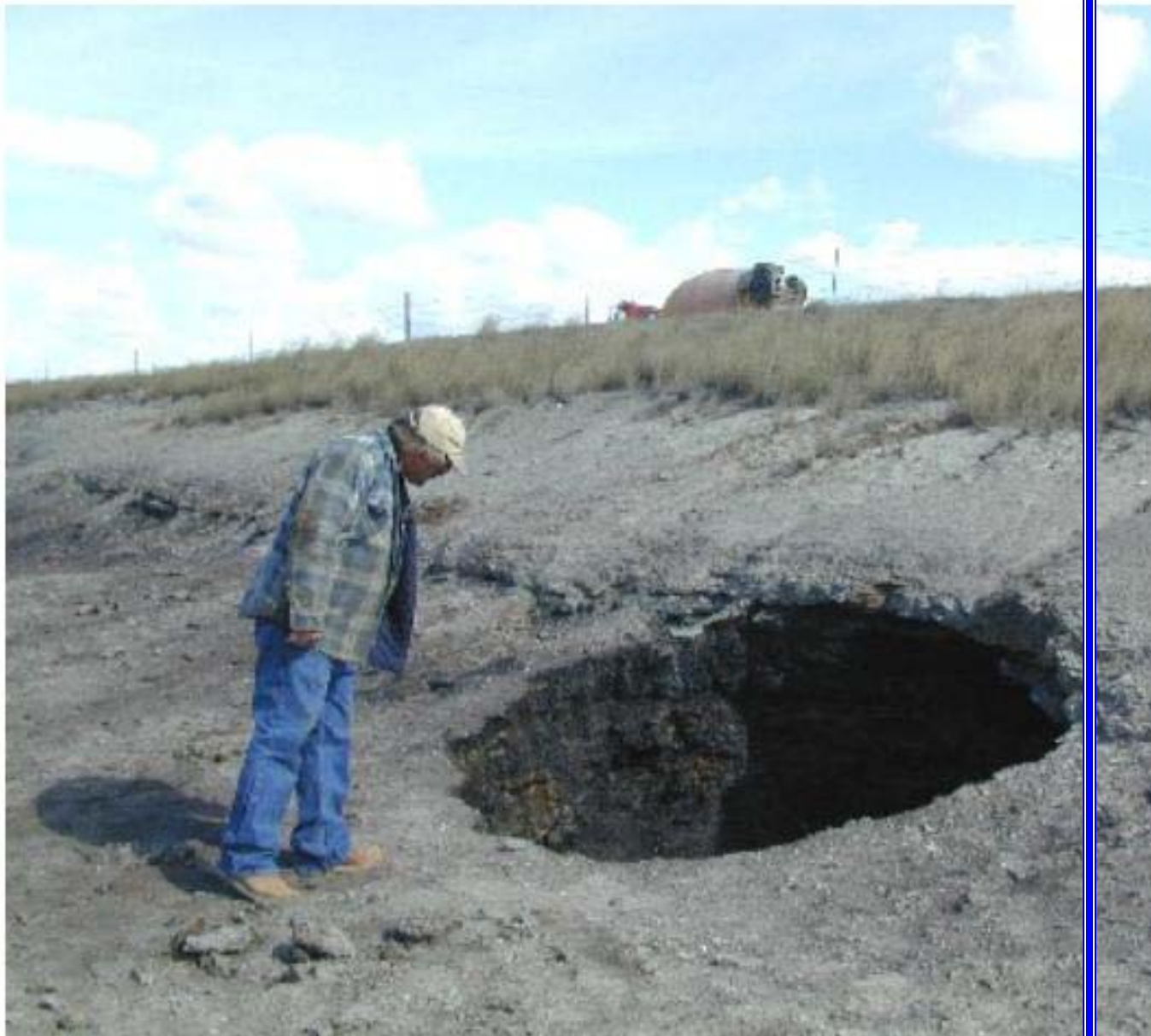
This fifteen foot deep sinkhole was located on the side slopes of an old land fill now owned by Willard Schnell. It was within 75 feet of Lehigh Road.
