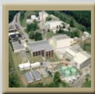
HFIR Second Cold Source and Guide Hall
