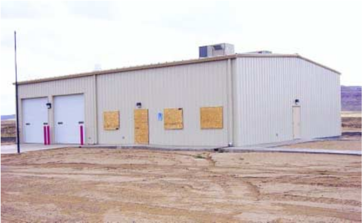
Front View of Hopi Wildland Fire / EMS Station in Kykotsmovi, Arizona.
