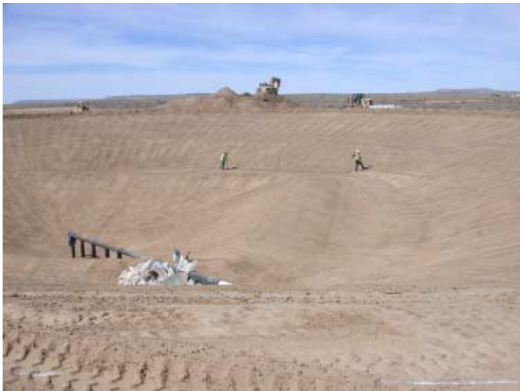
Kykotsmovi Sewage Lagoon Public Facility Project – Pond Construction.
