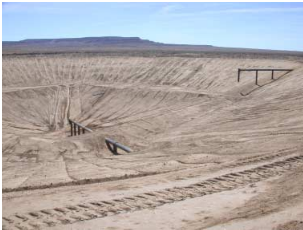
Kykotsmovi Sewage Lagoon Public Facility Project – Pond Construction.
