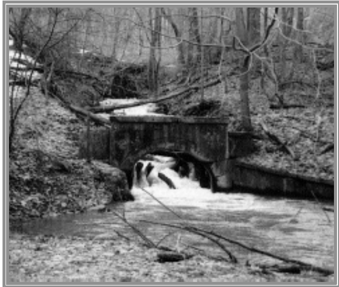
Hoffman Tunnel Underground Mine Drainage
