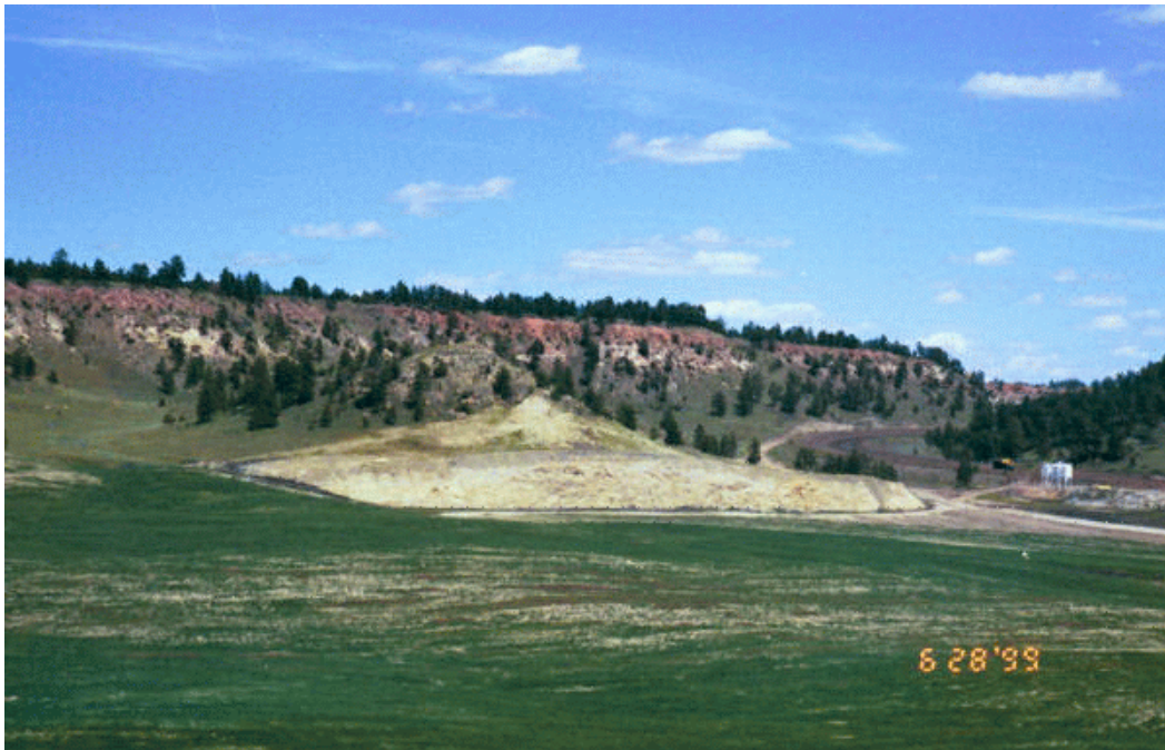
(Unapproved Bluff Extension feature constructed by Peabody Big Sky Mine)
