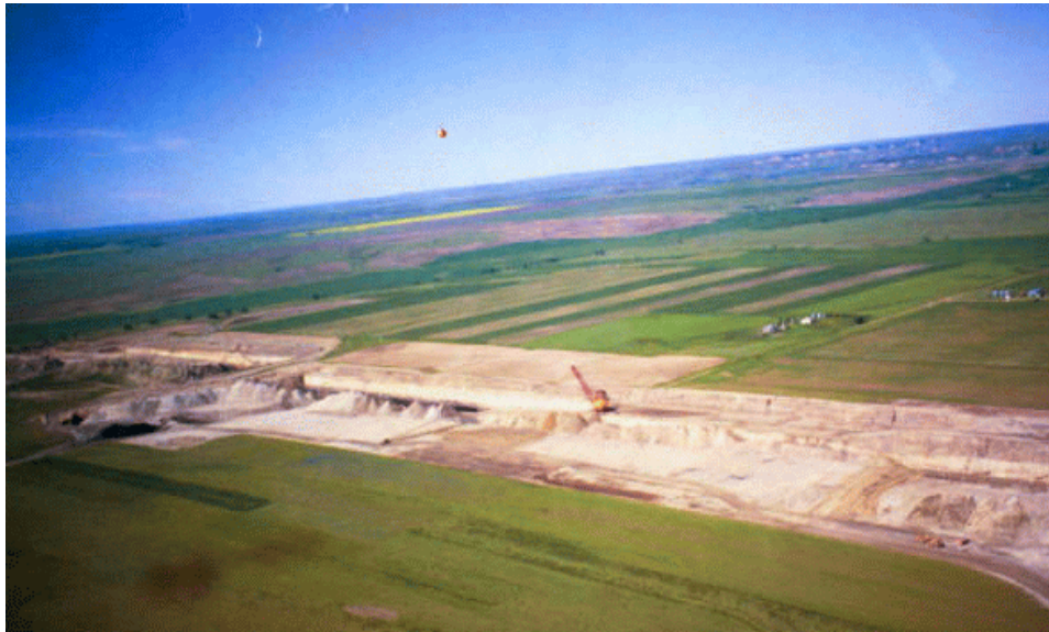
(Contemporaneous mining progression from farming to mining to reclamation and farming again) (at the Knife River Coal Company Savage mine)
