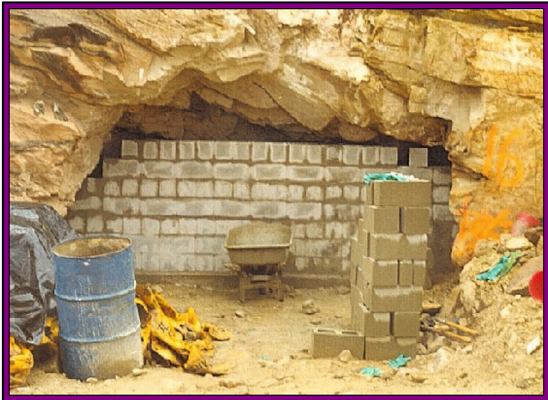
Portal being sealed with concrete block & rebar at Carrizo-1.
